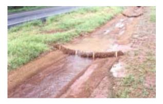
Figure 9 Vegetated waterway construction with woven coir mats and coir wattles.
