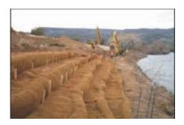
Figure 6 Soil lift construction with coir block system.
