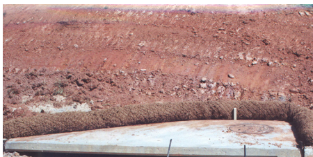
Picture 3. Coir wattle placed on the slope above curb inlet
