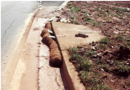
Picture 3. Coir wattle placed on the slope above curb inlet
