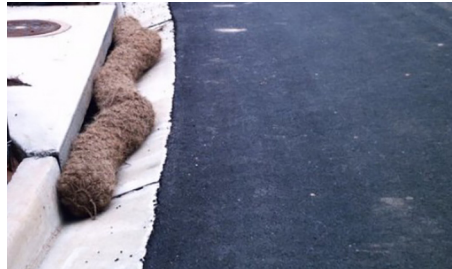
Picture 2. Coir wattle placed with coir twine loops
