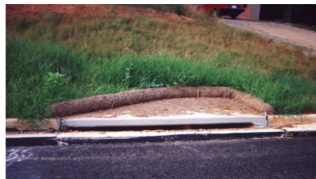
Picture 3. Coir wattle placed on the slope above curb inlet
