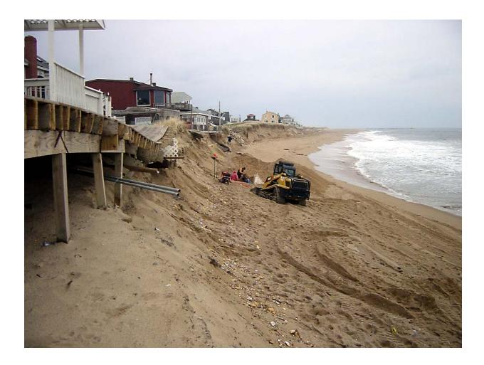
The erosion of beach and dune that has been occurring immediately north of the center parking lot groin now directly threatens public infrastructure as well as private property. The current effort to reinforce the area consists of the placement of a "soft" biogradeable structure to buttress the remaining dune. While It does not solve the erosion problem, it should greatly reduce the loss of sand from the dune during storms.
