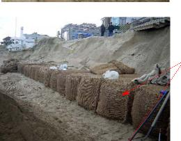
December 2, 2008, several additional tubes have been placed and a second team has started to the north constructing bags in a southerly direction. The second layer of tubes have been placed. These are 6 foot long and have been placed at a right angle to and on top of the tubes shown in the proceeding pictures.
