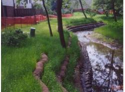
As a result of the initial success of Phase I, Phase 2 of the project, which will involve stabilizing another 850 ft. section of the streambanks with the coir block and fabric system, is scheduled to be constructed beginning fall of 2004. For more information, contact Gray at 630-261-1133 or <a href="mailto:TedGray@msn.com">TedGray@msn.com</a> or www.streamandlakerestoration.com.
