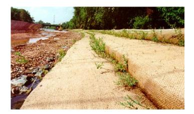
Figure 1: Bioengineered river bank stabilization, an innovative fabric-encapsulated technique.
