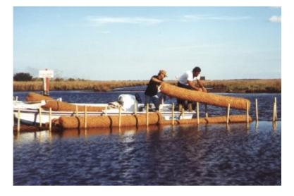
Figure 2: Use of coir rolls in shoreline stabilization.
