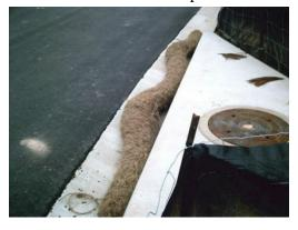
coir decays at a much slower rate, holds it shape and structure for a longer time and wildlife won't eat it." One of the company's biodegradable sediment control products, BioD-SiltCheck<sup>TM</sup>, functions as a check dam. It features a coir fiber log body, which filters and reduces the speed of flowing water. Available in 9-in. or 12-in. sizes, this body is connected to two coir filter aprons on either side and is placed perpendicular to the flow. The upstream
