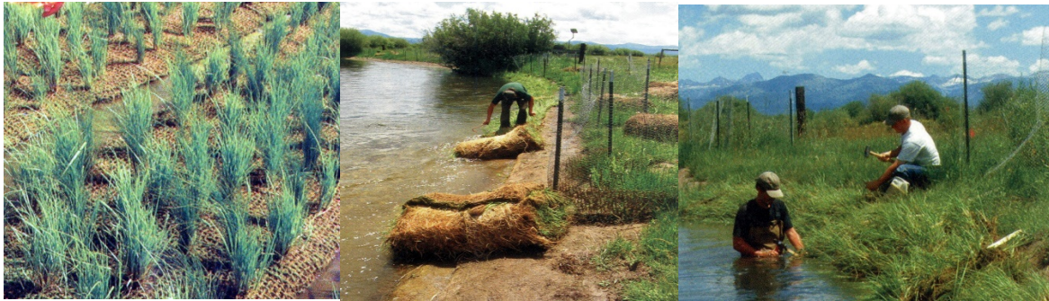
Restoring eroded wetland with vegetated coir pillows.
