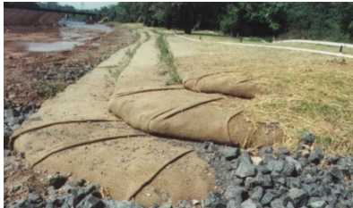
Streambank restored with vegetated soil-lifts
