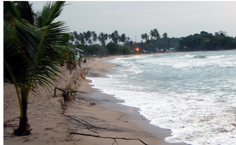
Severely eroded beach
