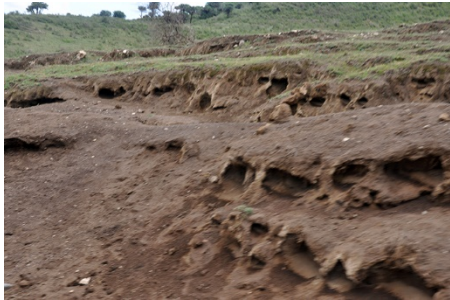
Severely eroded slope
