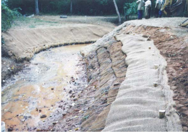
Figure 2. Upon completion of construction
