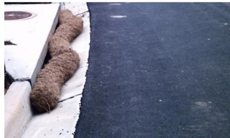
**Picture 3. Coir wattle placed on the slope above curb inlet**
