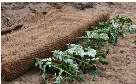
Figure 3. Improved coir block system with planting holes.
