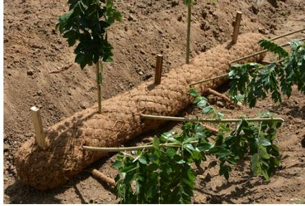
Figure 4. BioD-SuperRoll 12 with invisible planting holes.
