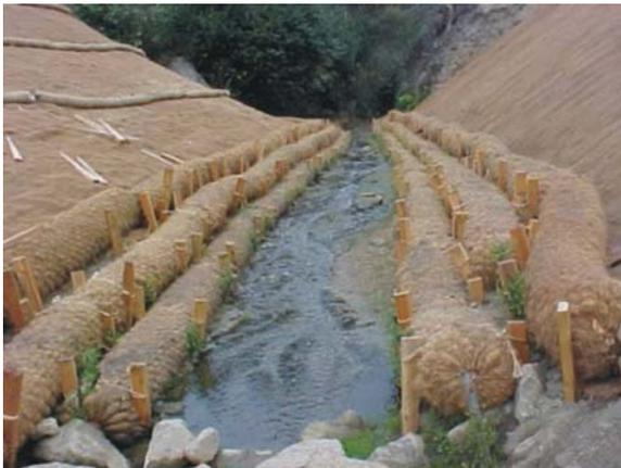
**Figure 2 Densely-packed coir logs placed on a stream.**
