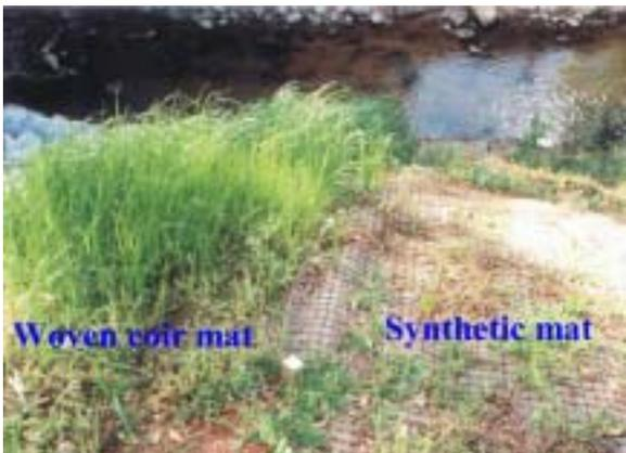
**Figure 4 Vegetation is coming through a woven coir mat better than a synthetic permanent mat.**
